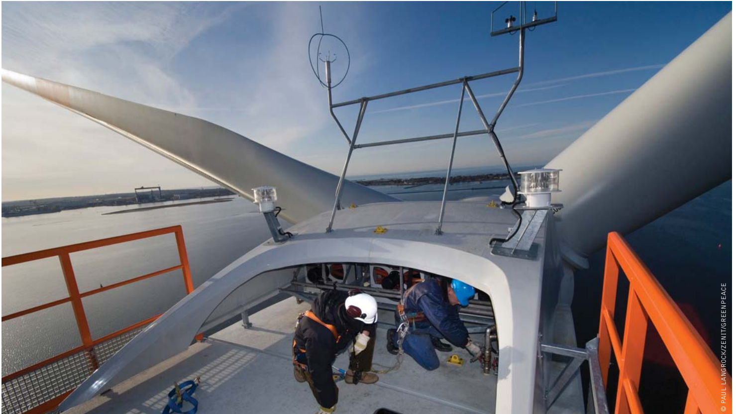
image TEST WINDMILL N90 2500, BUILT BY THE GERMAN COMPANY NORDEX, IN THE HARBOUR OF ROSTOCK. THIS WINDMILL PRODUCES 2,5 MEGA WATT AND IS TESTED UNDER OFFSHORE CONDITIONS. AT LEAST 10 FACILITIES OF THIS TYPE WILL BE ERECTED 20 KM OFF THE ISLAND DARSS IN THE BALTIC SEA BY 2007. TWO TECHNICIANS WORKING INSIDE THE TURBINE.
